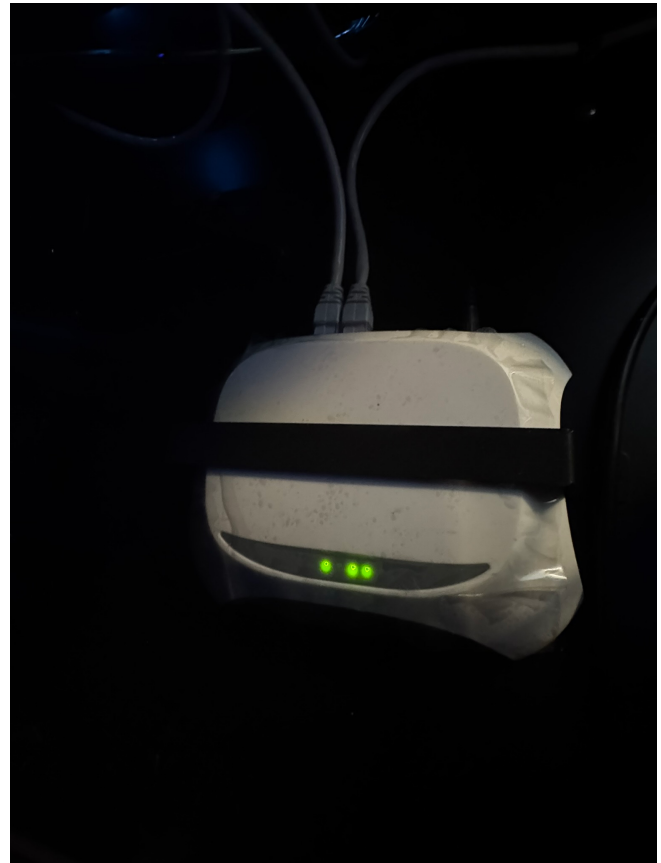
Figure 13: Router power and ethernet cables (some machines have the ethernet cable connected directly between the PC and motion controller underneath the seats)
